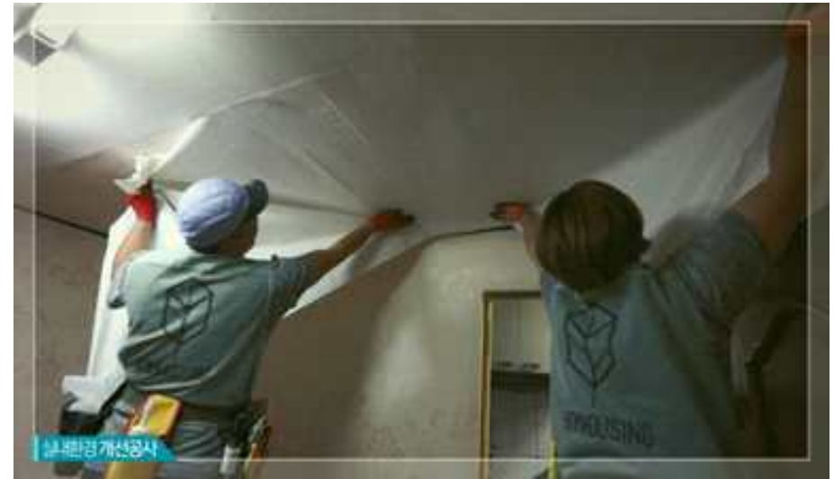
Application of eco-friendly wallpaper on old house
