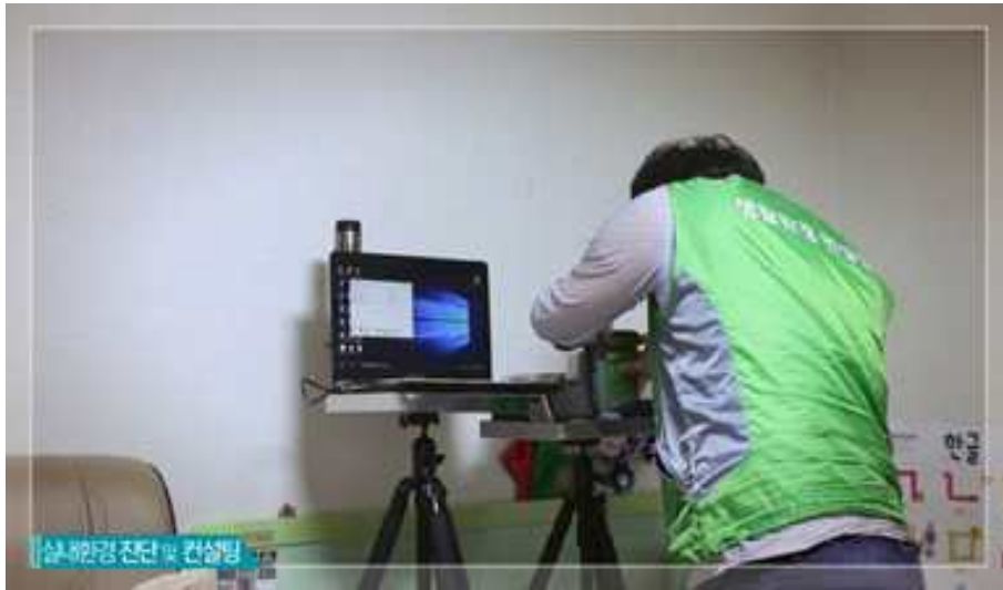
Indoor Air Quality Monitoring Equipment
